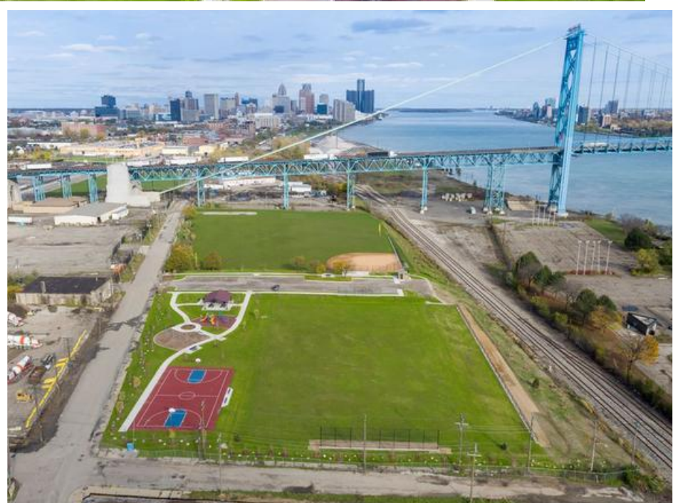
Riverside Park Phase 1 Detroit, MI.
